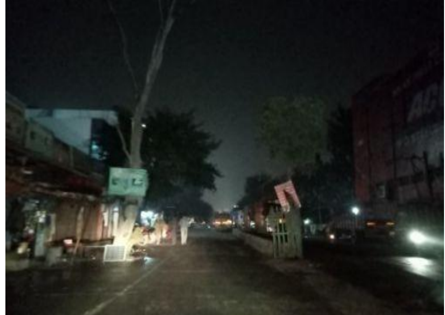
Non-functional street lights at Transport Nagar road
