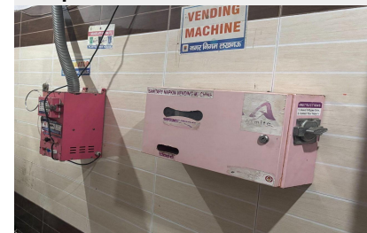
Hand dryers and sanitary napkins dispenser
