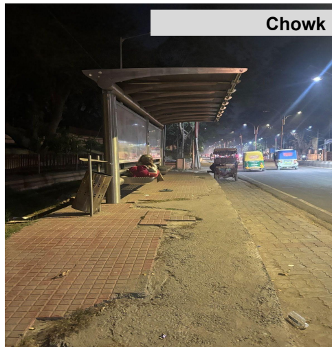
Broken pavers lacks maintenance
